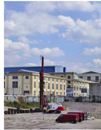
Driving of a sheet pile curtain using a Vibrodriver @20RHFV
